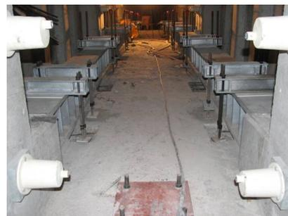
Fig. 5 Strengthened box girders' bottom slab
