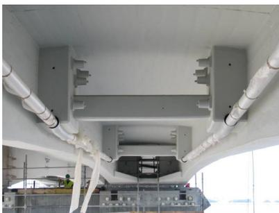
Fig. 4 External pre-stressing of the deck
